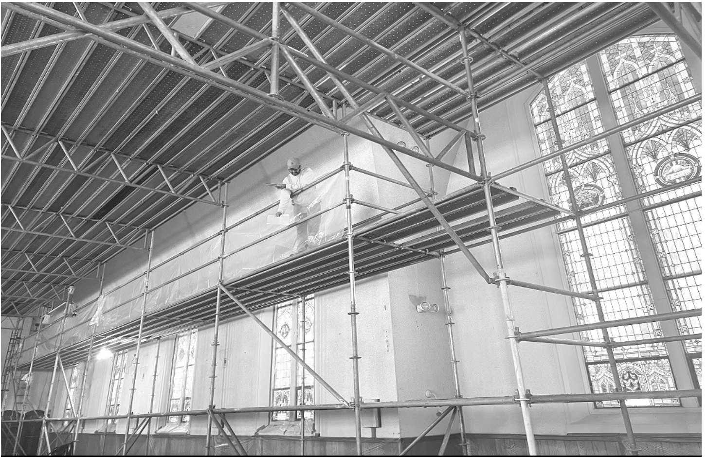
Scaffolding setup at the Historic Church is now complete. ▲ Work begins on the walls and ceiling repairs, skim coating, and painting. ▼
